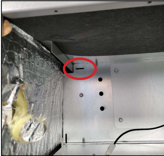
Figure 12. Notch for Control Panel Relocation
